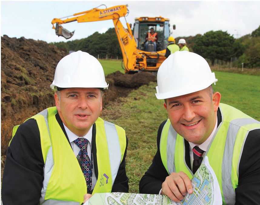
Ground breaking: Sedgefield Borough Homes (sbh) chief executive Colin Steel (left) with Neil McMillan, director of Carillion Developments
